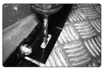
NOTE - Beware of electric cables when drilling holes
