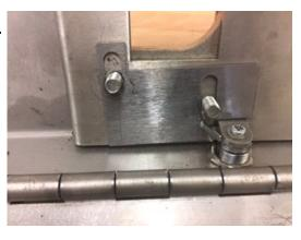
Now fit the nuts & washers and tighten to about 5 Nm then slacken the pawl & claw bolts (right on photo) by ¼ turn to allow them to move freely.
