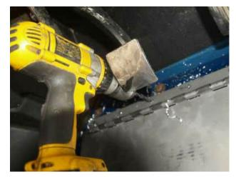
of three screws is sufficient. Insert screws into the holes with washers, then screw on a security nut & washer on to each. The hexagonal portion of the nut must face downwards. Make sure you are happy with its operation before you fully tighten.
